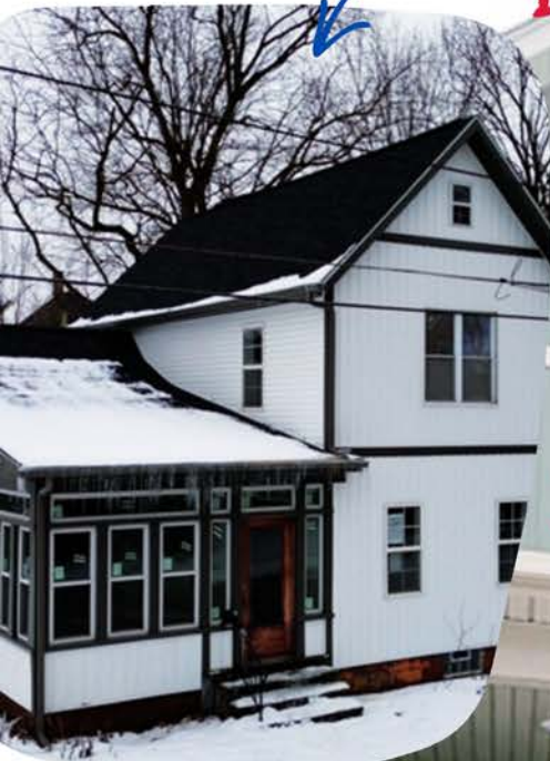
Renovation of a 19th century home on 7th St. NW
